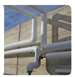
Insulock PVC cladding is a complete insulation system. The Insulock Fitting Cover System consists of one piece pre moulded high impact PVC fitting covers which include elbows, tee/valves, end caps, mechanical line couplings, specialty fittings, white and indoor colour jacketing.
